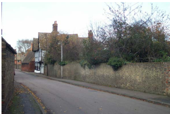
Boundary wall to The Gables
